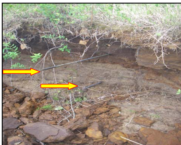
Figure 13. Photograph of exposed bank pins.
