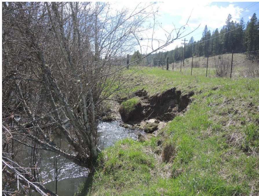
Figure 18. Site 5 Before Work Started
