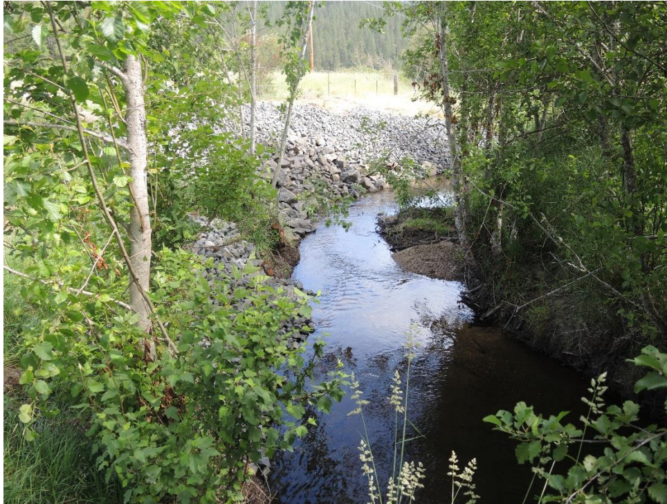
Figure 19. Site 5 After Work Completed
