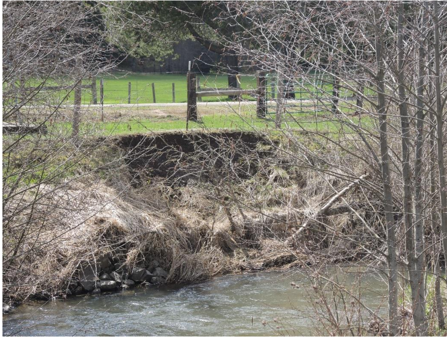
Figure 5. Site 2 Before Work Started
