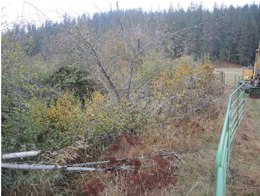
Figure 8. Site 3 Before Work Completed
