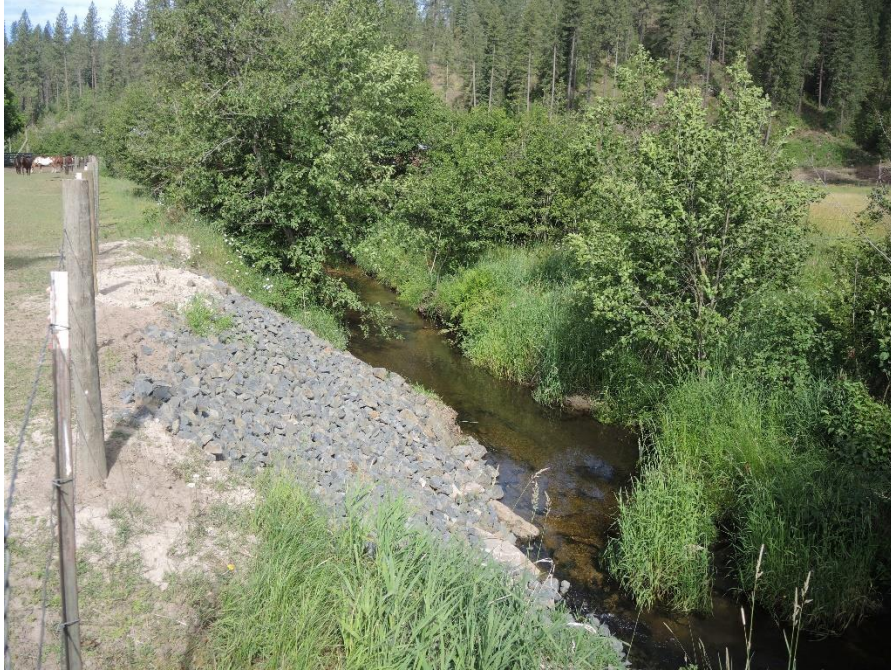
Figure 7. Site 2 After Work Completed
