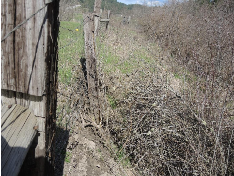
Figure 13. Site 4 Before Work Completed
