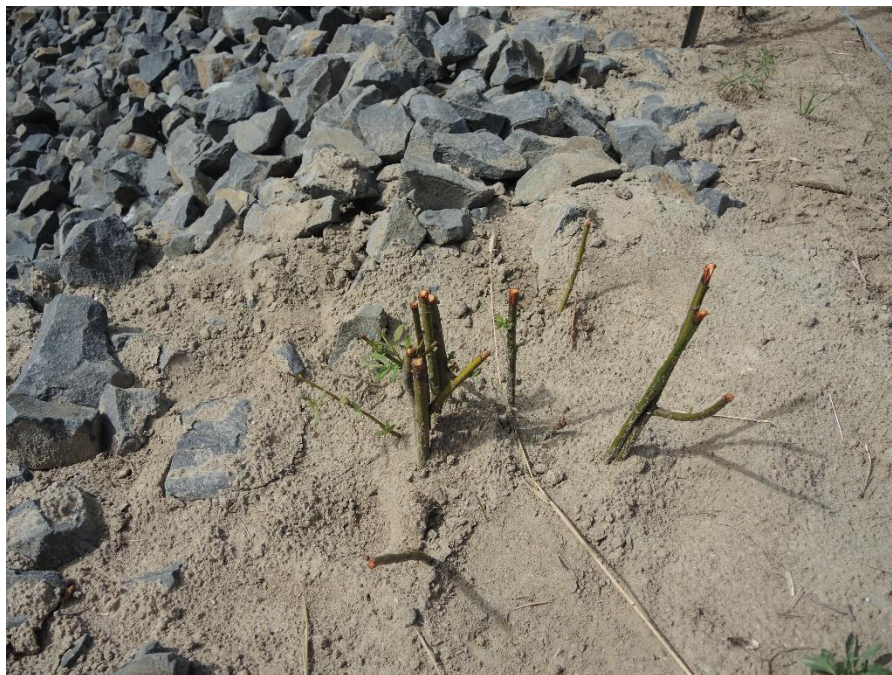
Figure 22. Site 5 After Work Completed. Willows planted
