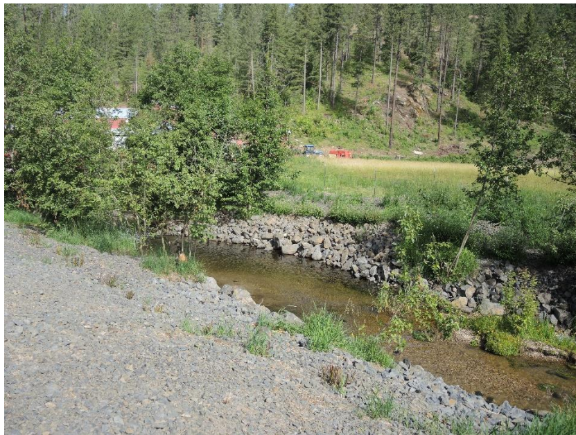
Figure 4. Site 1 After Completed Work
