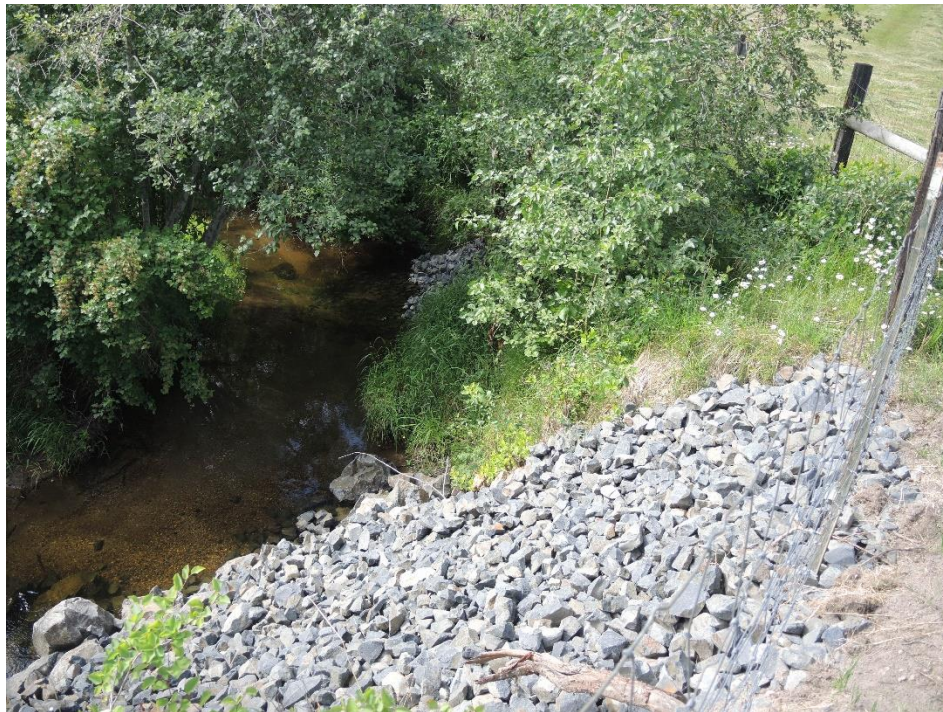
Figure 16. Site 4 After Work Completed
