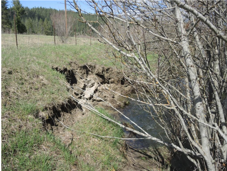
Figure 17. Site 5 Before Work Started
