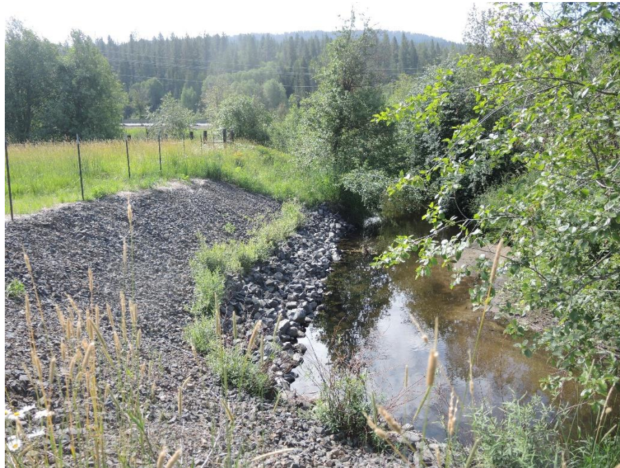
Figure 12. Site 3 After Work Completed
