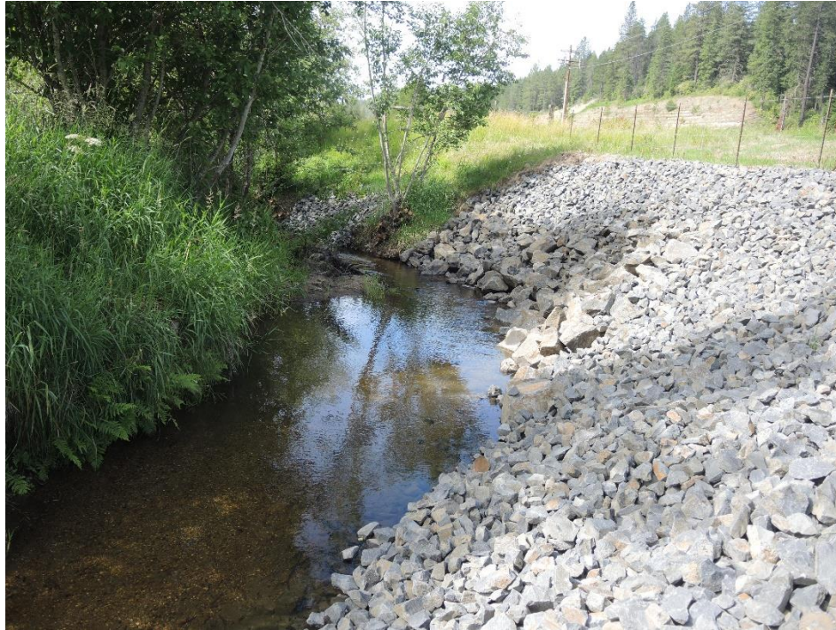
Figure 21. Site 5 After Work Completed
