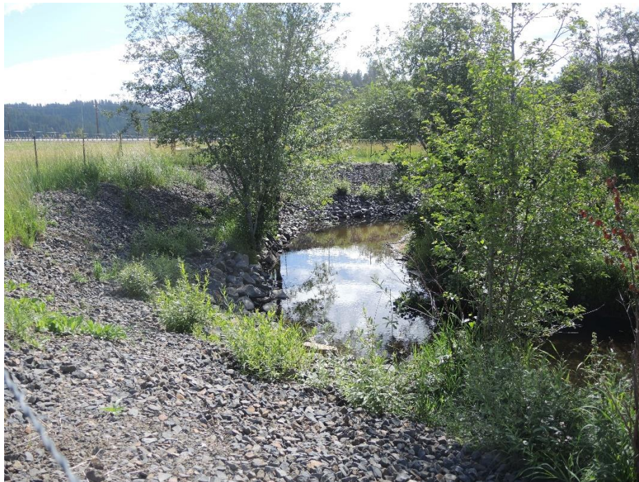
Figure 10. Site 3 After Work Completed
