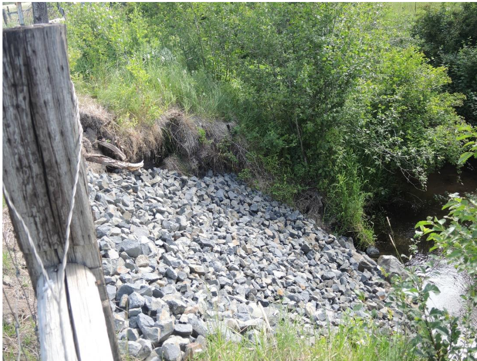
Figure 14. Site 4 After Work Completed
