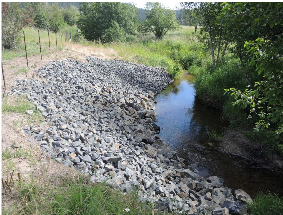
Figure 20. Site 5 After Work Completed
