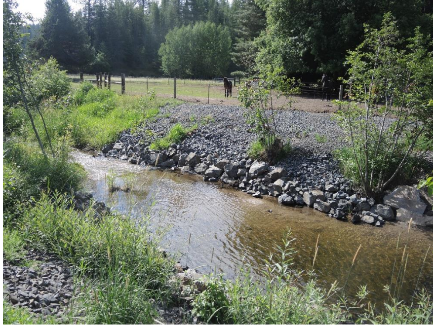
Figure 3. Site 1 After Completed Work
