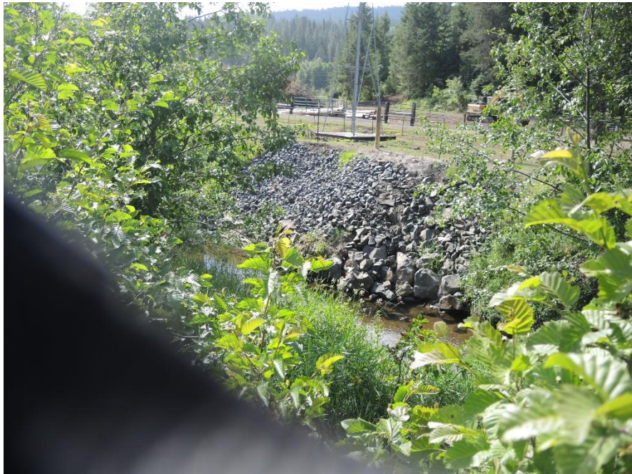
Figure 6. Site 2 After Work Completed
